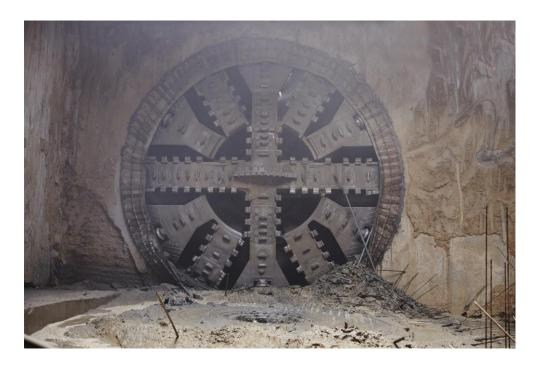
The JV uses a total of two (2) TERRATEC TBMs for the execution of the tunnelling works between Jama Masjid and Kashmere Gate Stations. The Tunnel Boring Machine emerged at Lal Quila Station site after making a 1,351m long tunnel from Kashmere Gate Station. A total of 967 rings have been inserted concurrently along with the tunneling process. Another TBM is working on a 1,356m long tunnel on the down line.
